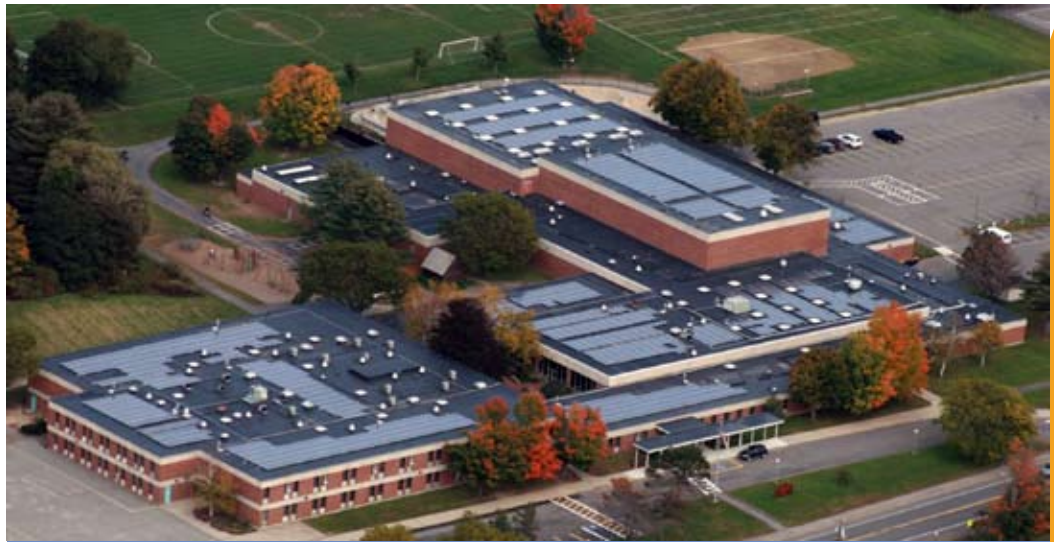
City of Newburyport's municipal solar project. Spread over three facilities the 502kW system is comprised of 2,184 230w panels. The photovoltaic system's power output is equivalent to 70 homes and will offset 402 tons of carbon output per year.
