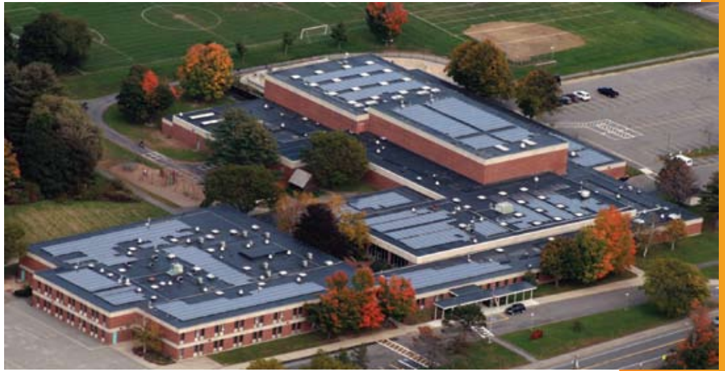
City of Newburyport's municipal solar project. Spread over two facilities the 502kW system is comprised of 2,184 230w Canadian Solar panels. The photovoltaic system's power output is equivalent to 70 homes and will offset 402 tons of carbon output per year.
