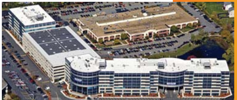
Cummings Properties' flagship green office building, the TradeCenter128. Over 1000 Canadian Solar panels reside on the parking garage roof and supply over 200kW to the 500,000 sqft LEED Gold certified office building
