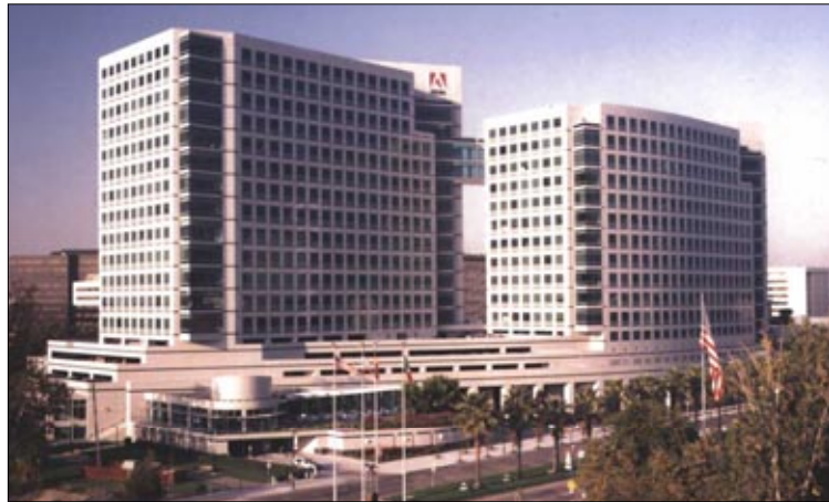
At their headquarters, Adobe Systems equipped 3,400 workstations with Isolé to reduce their plug load energy consumption.
